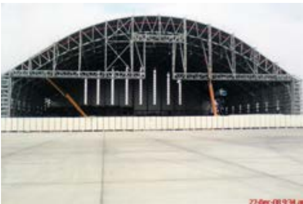
Project: Gamco Hangar, Abu Dhabi, UAE
