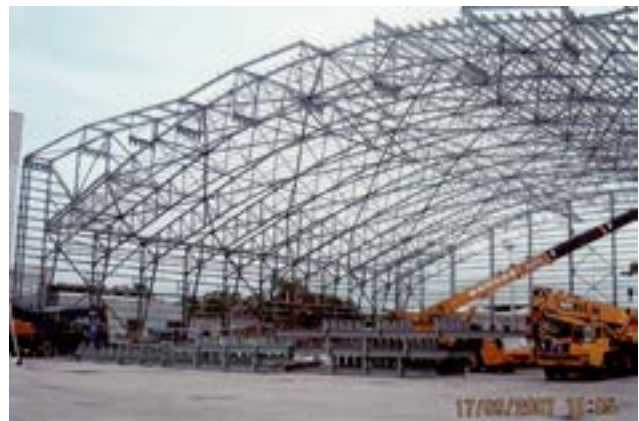
Project: Lufthansa Technik Hangar, Philippines
